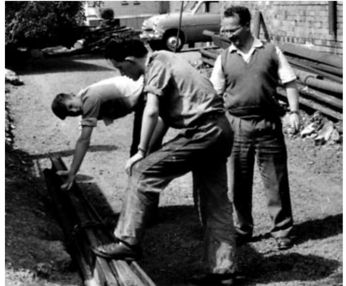
*Ian Stewart (right) supervises Ollie Scott (hand on rail) and Ian Jenner, laying a turnout behind the pump house to connect temporary tram storage tracks c.1965.*
