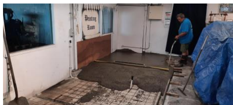
Above: Half-way through the concrete pour.
