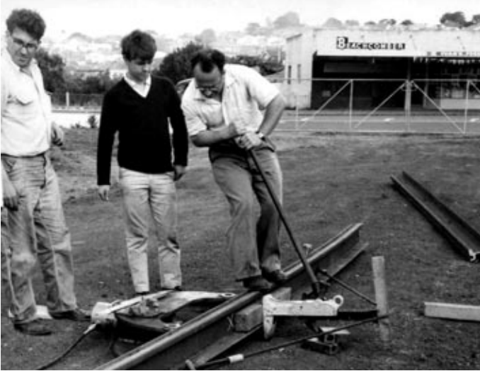
Ian leans on the operating bar of a home-made rail bending jack to correct over-bending by the hydraulic jim-crow (seen on the other side of the rail) watched by Ian Mison (left) and Kevin Swan. c. 1965.
