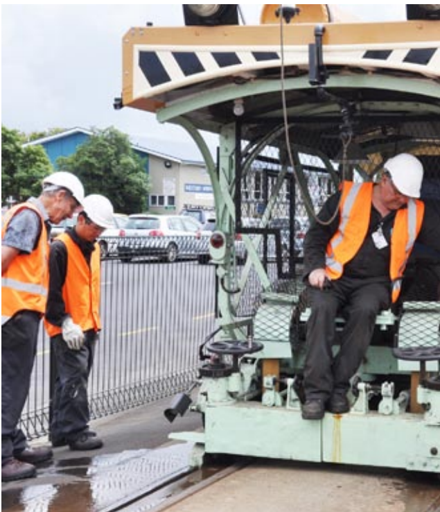
Noel Ashley is in the driving seat as the grinder reprofiles a section of track alongside Motions Road, observed by Tony Messenger (left) and Leyton Chan.
