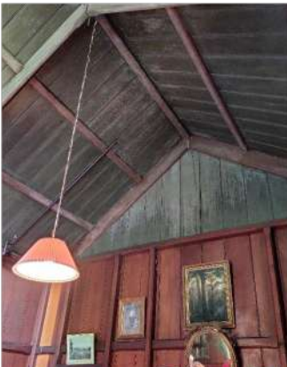
INTERIOR front room
