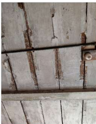
INTERIOR ceiling lean-to
