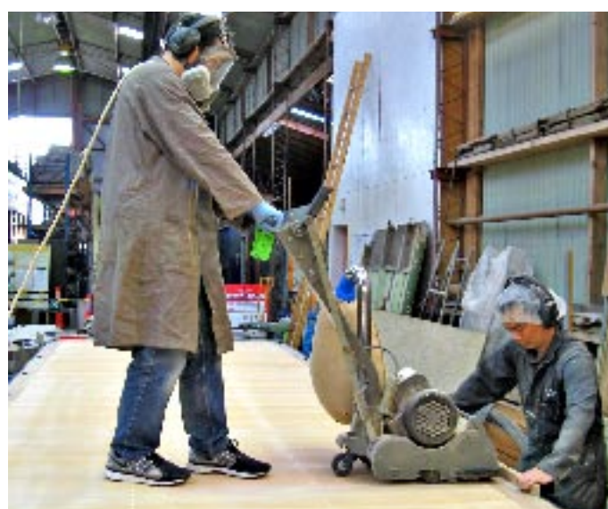
Vincent Chan (left) and twin brother Leyton sanding the floor of trailer 21.
