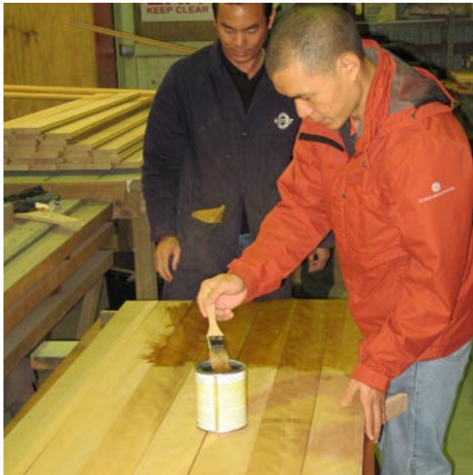
New member Zam Yang seals the new kauri floor boards for trailer number 21 with shellac, closely watched by project leader Leyton Chan.
