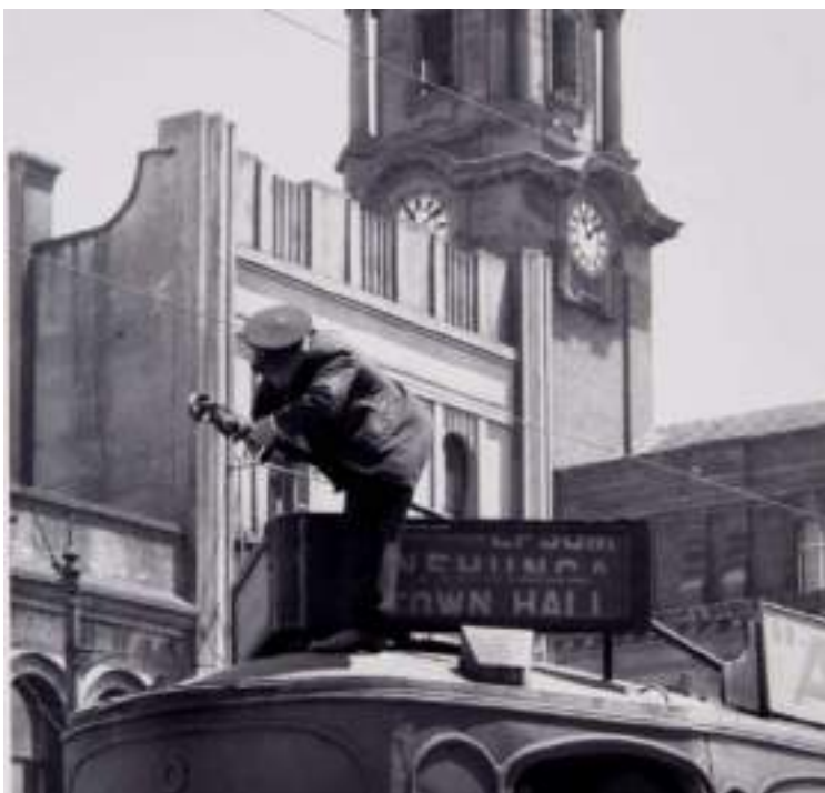
Above: Conductor on top of tram fixing tram pole. Lower Queen Street. Photo: Graham Stewart.
