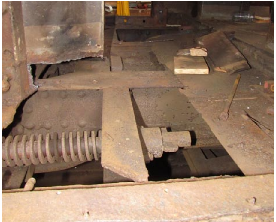
The drawgear springs exposed on carriage A1819 after rusty sections had been removed from an end vestibule as part of its restoration by Rail Section volunteers.
