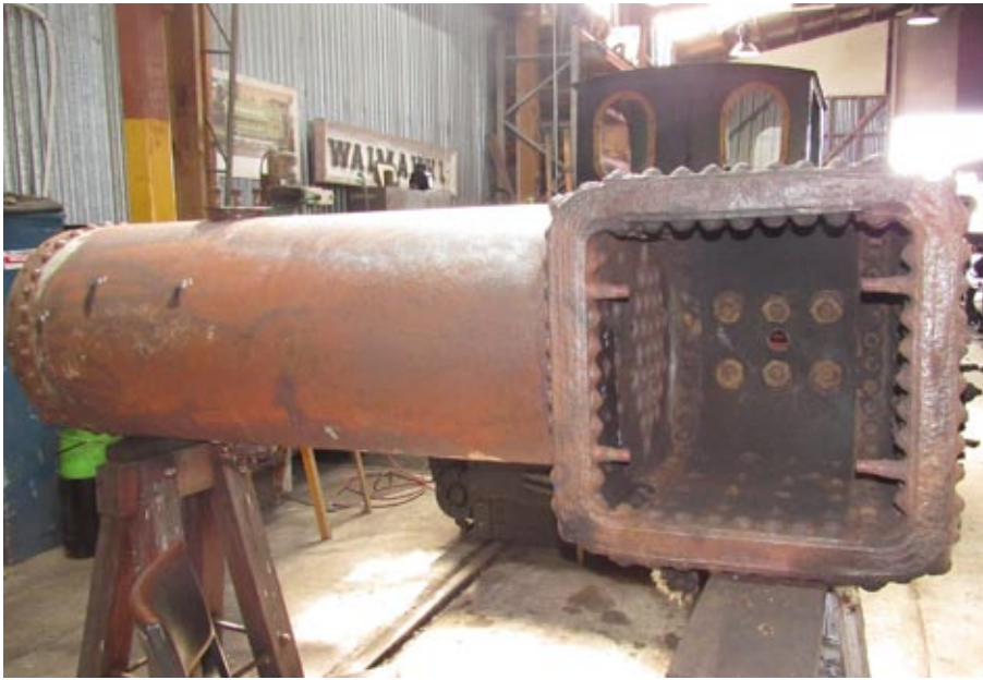
LEFT: The boiler of Bertha sits on its side on stands to enable a thorough inspection and the replacement of the boiler tubes and firebox.
