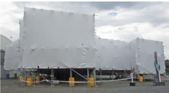
Protected from the elements, the Short Solent flying boat is wrapped in a cocoon of scaffolding and plastic.
